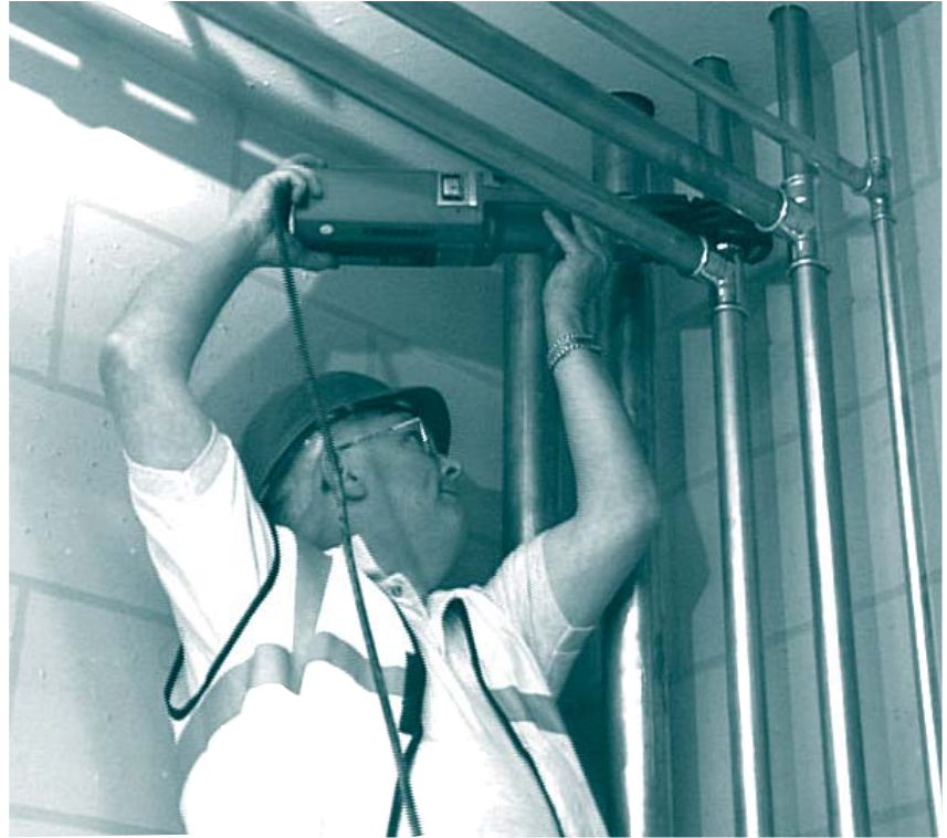
The new press fitting tool in action. The picture demonstrates the speed and ease of installation.
